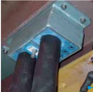
Driver's cabin: The Roxtec S 4x1 is used for mechanical anchorage of cables and reduced vibration.
